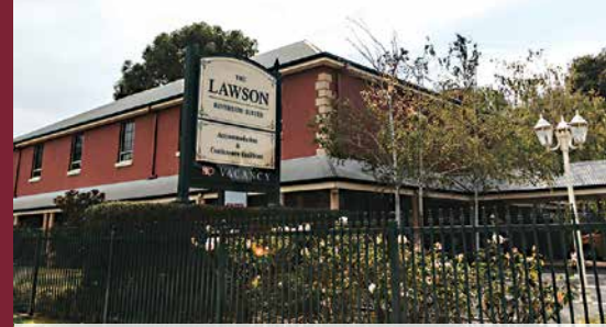
The Lawson Riverside Apartments
